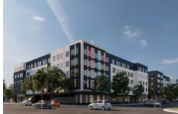
Broadway Station (140 affordable units)
