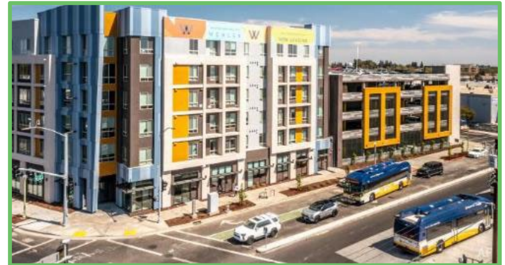
University/65th Street Station – 223 units
