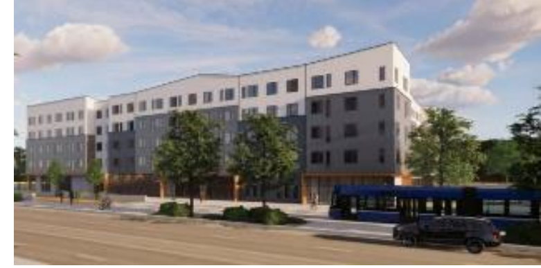
Arden/Del Paso Station (124 affordable units)
